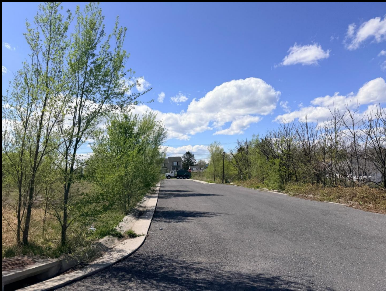
Collicello Street look toward Virginia Avenue
