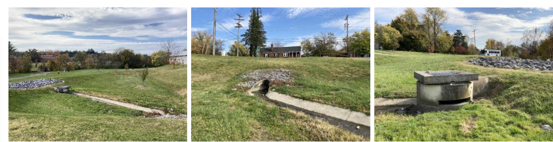
Existing Site overall photo looking SE (left), inlet with flowing water (middle) and existing outlet structure with signs of erosion on pipe (right)
