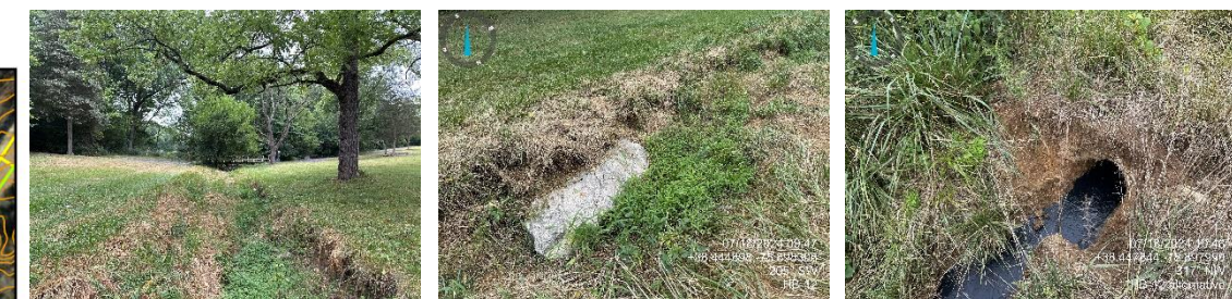
Existing Site photos demonstrating existing bank erosion and vegetation overgrowth as well as an unprotected culvert (right)
