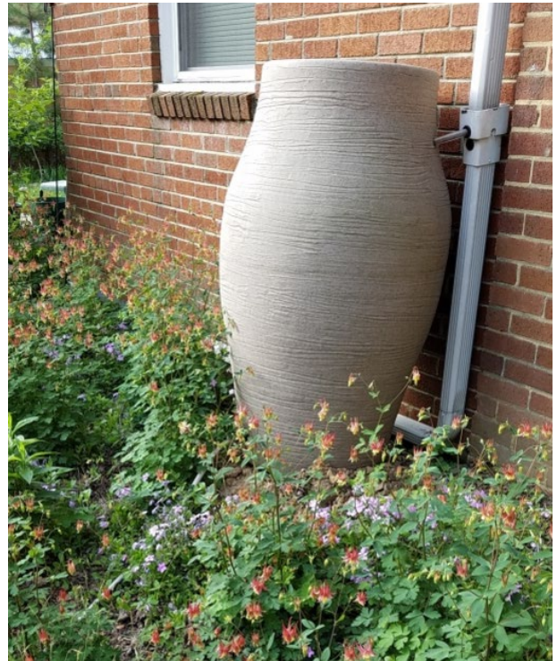
Rain barrels are a common residential BMP. They collect rain runoff from roofs, preventing the runoff from entering storm sewers. The collected water can be used to water plants.
