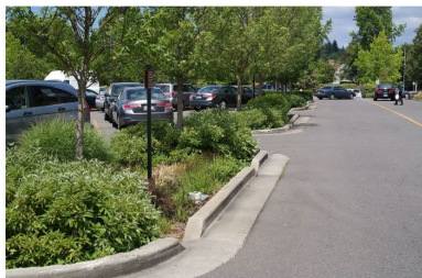
1. Terminal and interior islands help direct drivers, reduce driving speeds within parking lots and help reduce runoff.
