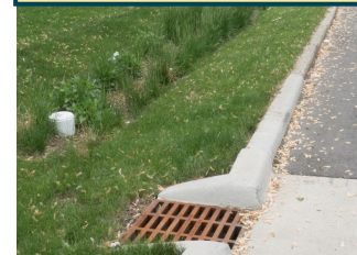
Bioretention/ Bioswale
