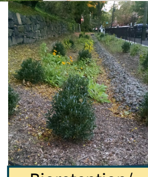
Bioretention/ Bioswale
