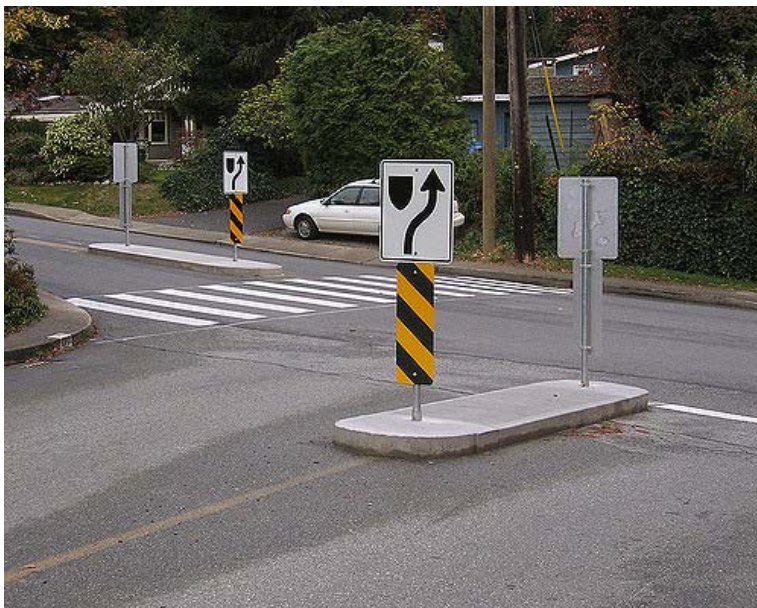
Traffic islands at stop sign
