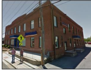
181 S Liberty St: Addition - Second Building on corner lot
