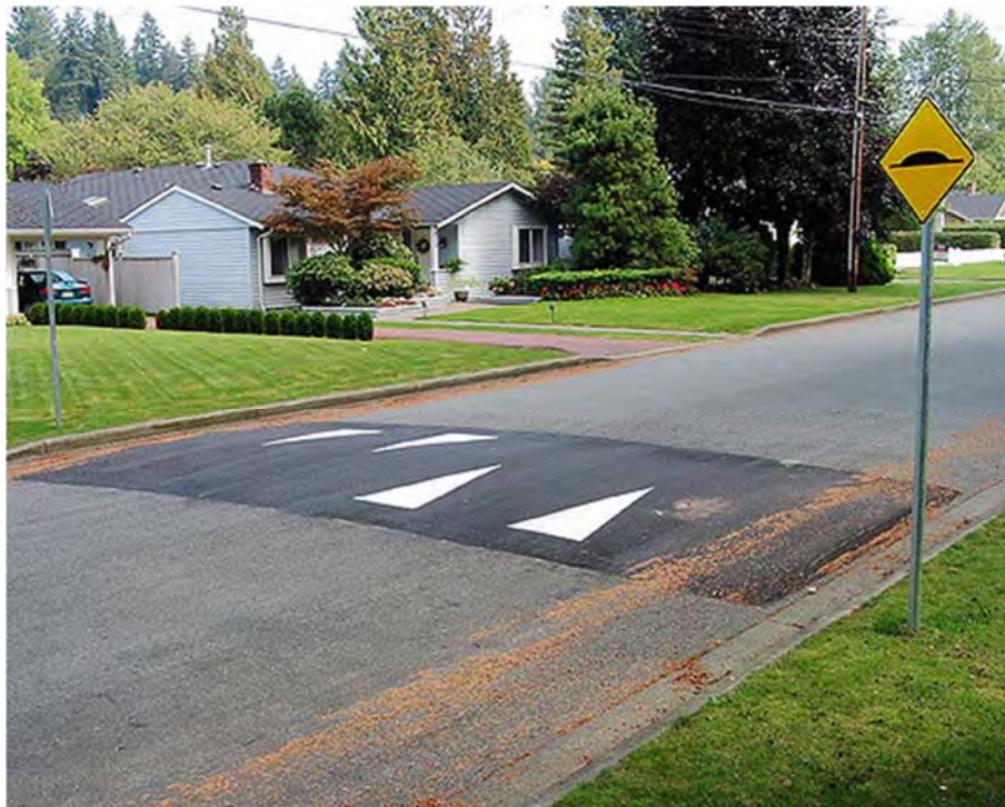
2) Speed Hump – wide traversable speed hump, approximately 6” tall
