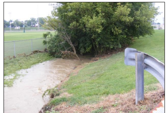
Locations throughout the City experience a range of flooding and drainage concerns. This site shows an interconnection of Blacks Run between the City of Harrisonburg and James Madison University.
