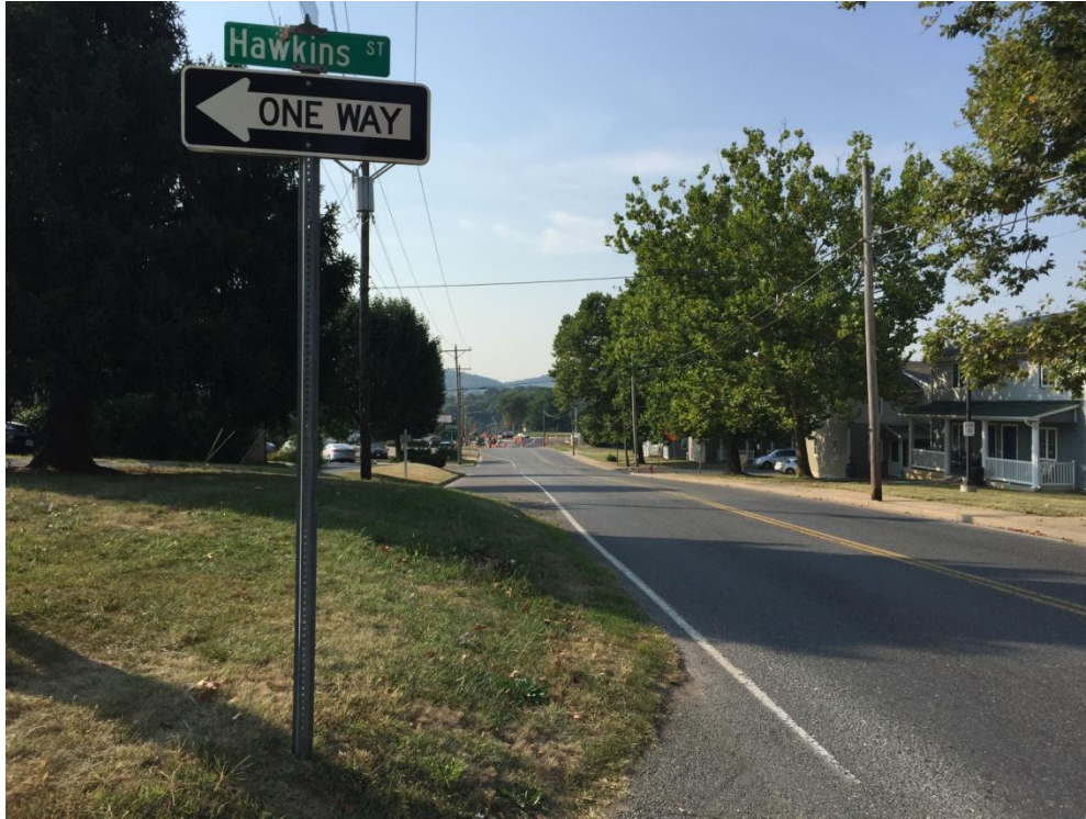
Figure 5. East side of Reservoir Street looking southbound towards Norwood Street. Future sidewalk to connect Hawkins Street residential street to future crossing improvements at Norwood Street.
