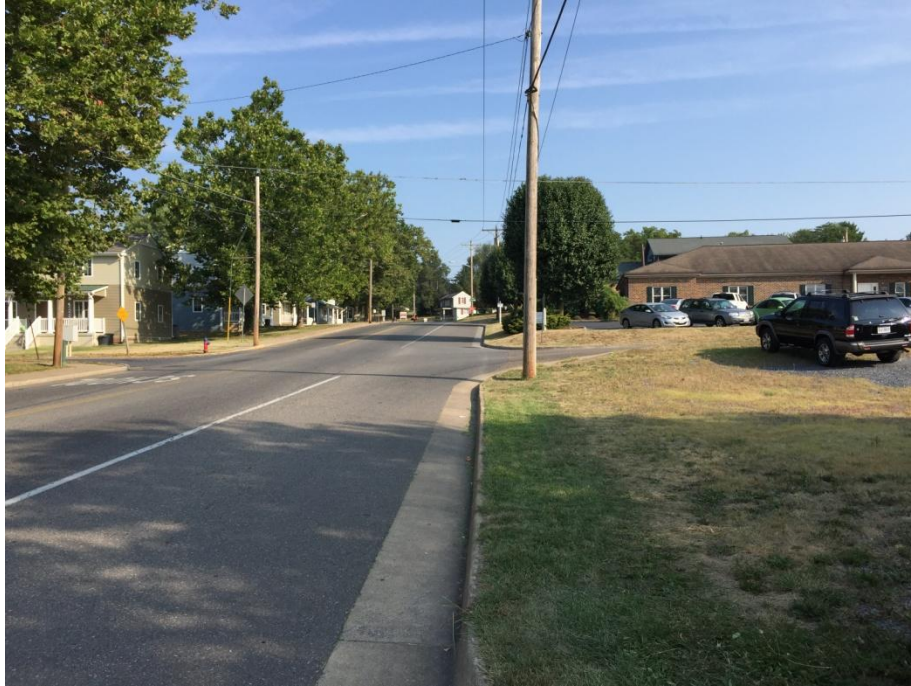
Figure 3. East side of Reservoir Street looking towards Norwood Street. Future sidewalk along Reservoir Street, and future crossing improvements at Norwood Street. Residential homes to the east and school is on the west. Students are currently crossing at this location.
