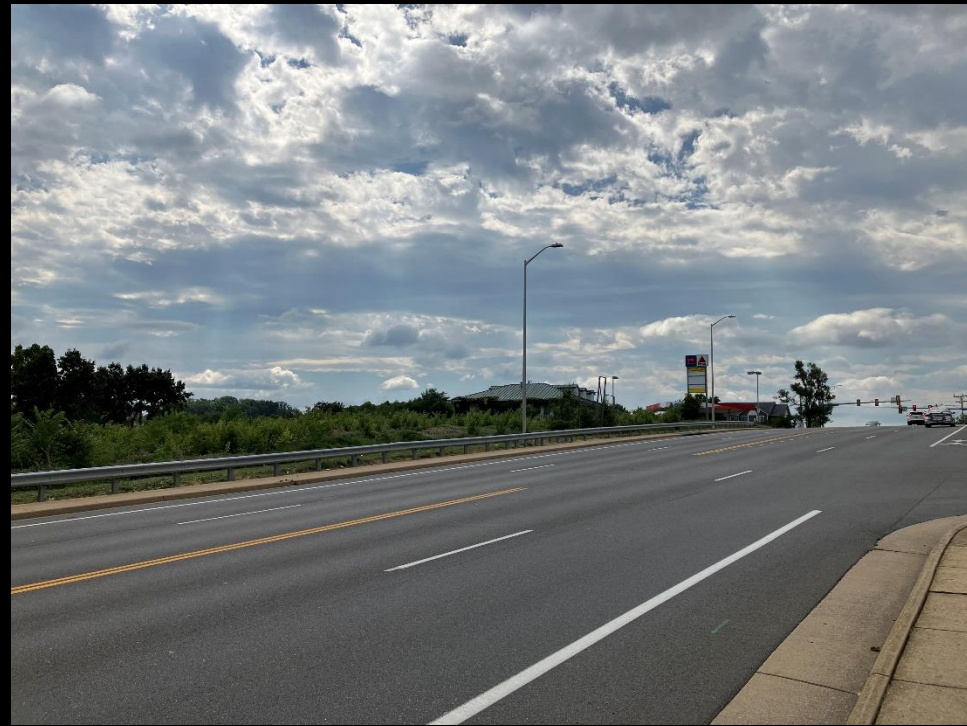
(above) On Port Republic Road looking uphill towards Devon Lane
