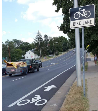
Bike lane signs complement pavement markings.
