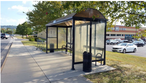
Bus stop shelter.
