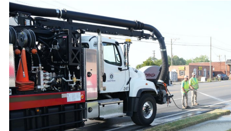
Storm Drain Cleaning
