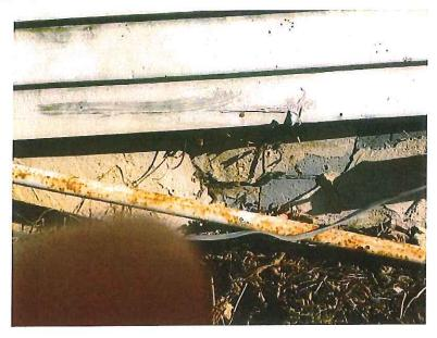
304.5 Foundation walls. All foundation walls shall be maintained plumb and free from open cracks and breaks and shall be kept in such condition so as to prevent the entry of rodents and other pests.
