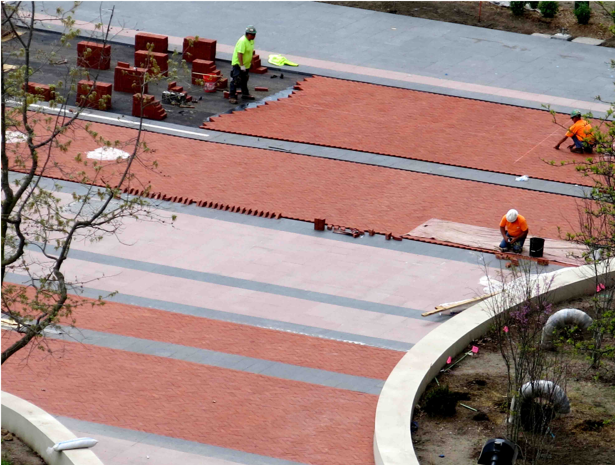
BANDED PAVING OF BRICK AND PAVERS AT COWLES COMMONS DES MOINES, IOWA
