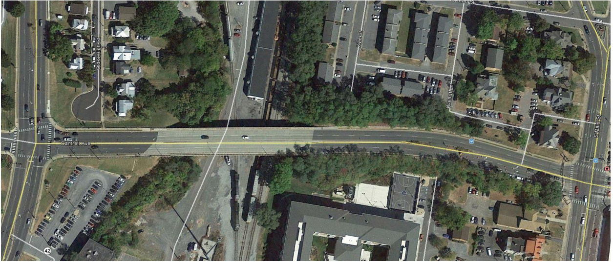
MLK Jr. Way Bridge Maintenance
