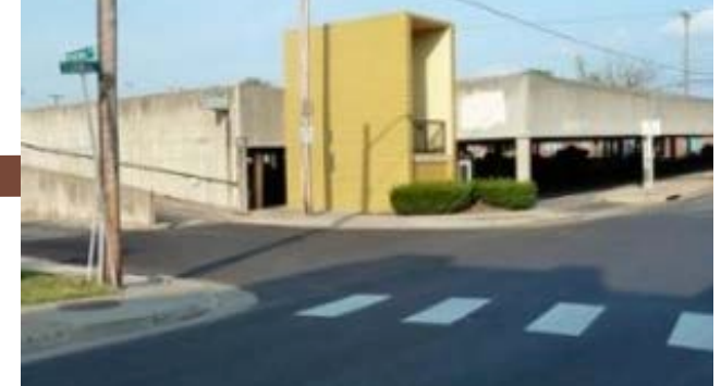
2013 – Parking deck built in 1971 on the corner of East Elizabeth and Federal Street
