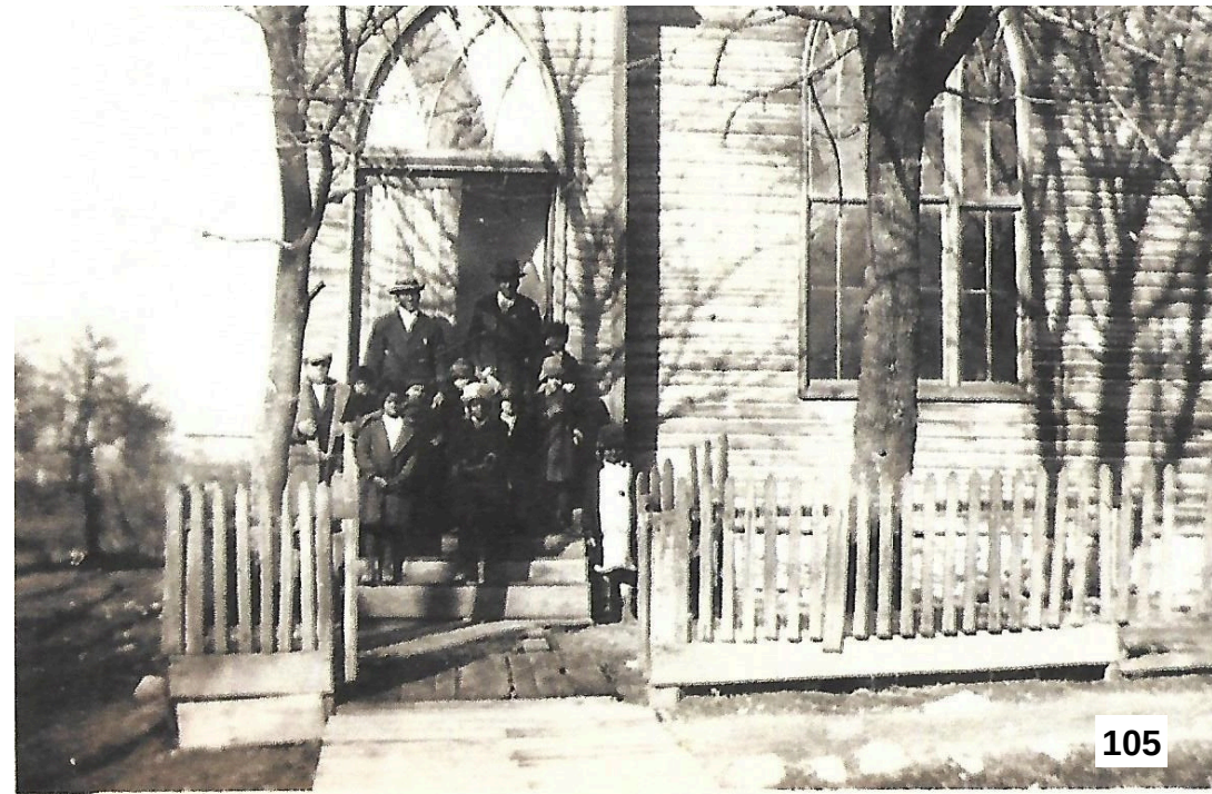
Kelley Street United Brethren in Christ Church , Source: NENA
