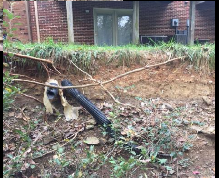
Exposed utilities and eroded streambank along Mountain View Drive
