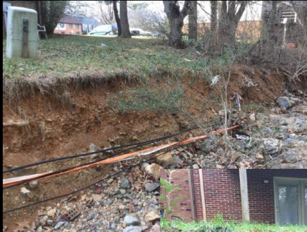
Exposed utilities and eroded streambank along Mountain View Drive
