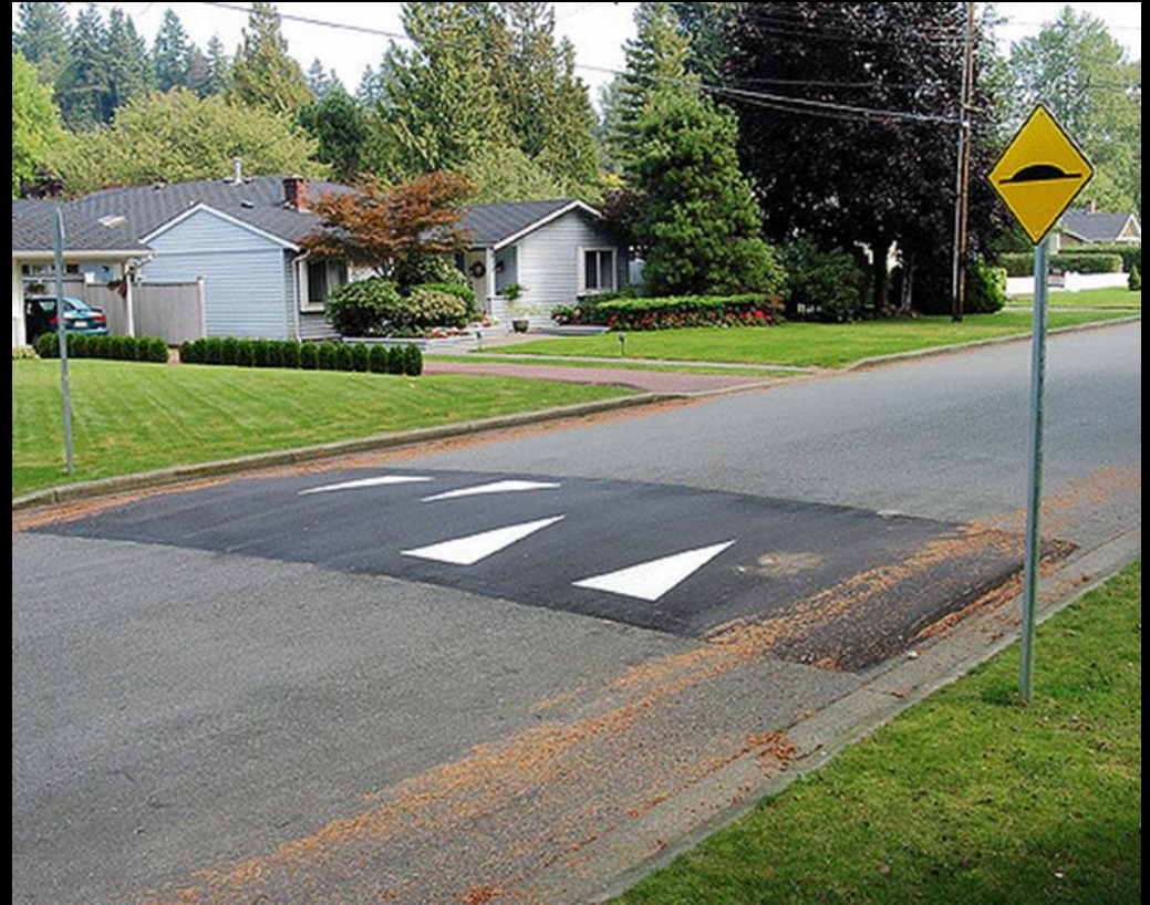
Speed Table – wide traversable speed hump, approximately 6" tall
