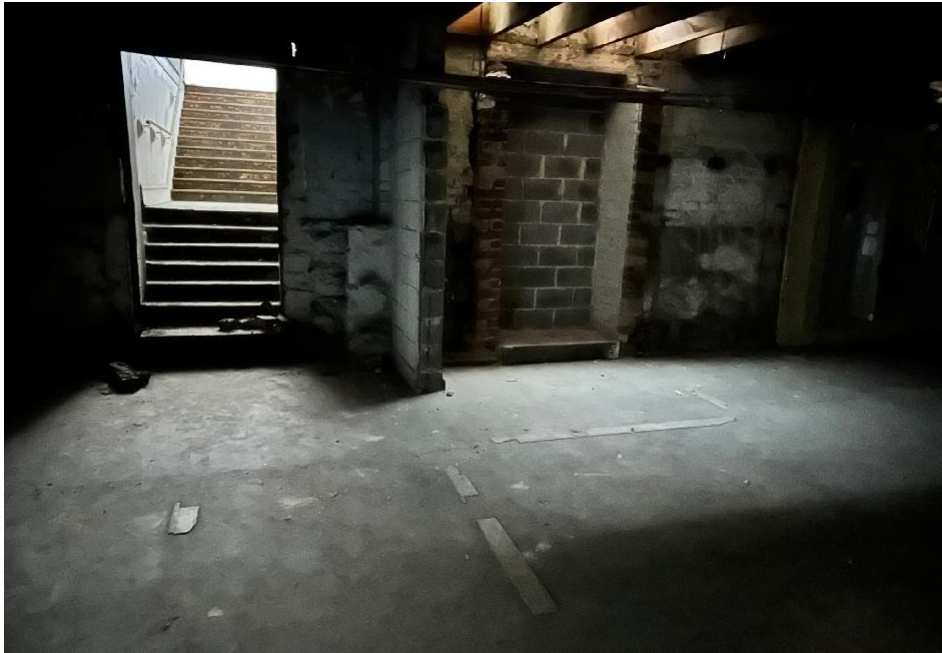
1879 BUILDING / STAIRS OF 1908 BUILDING
