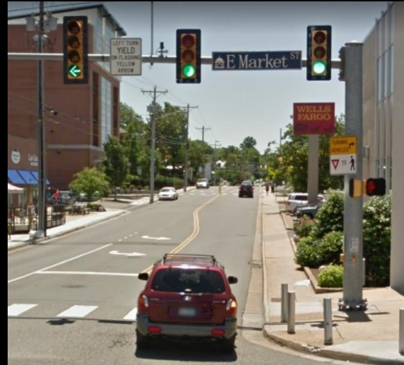
Leading pedestrian phase & "Turning Vehicles Yield to Pedestrians" signs
