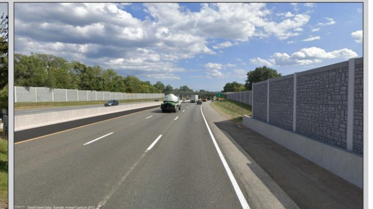
Example A - With Sound Barrier Wall
