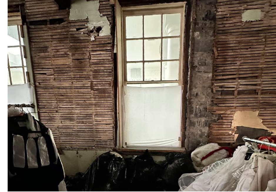
1908 BUILDING - EXTERIOR WALL
