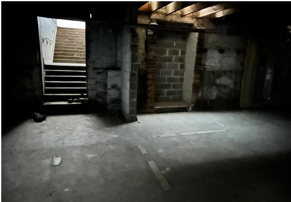
1879 BUILDING / STAIRS OF 1908 BUILDING
