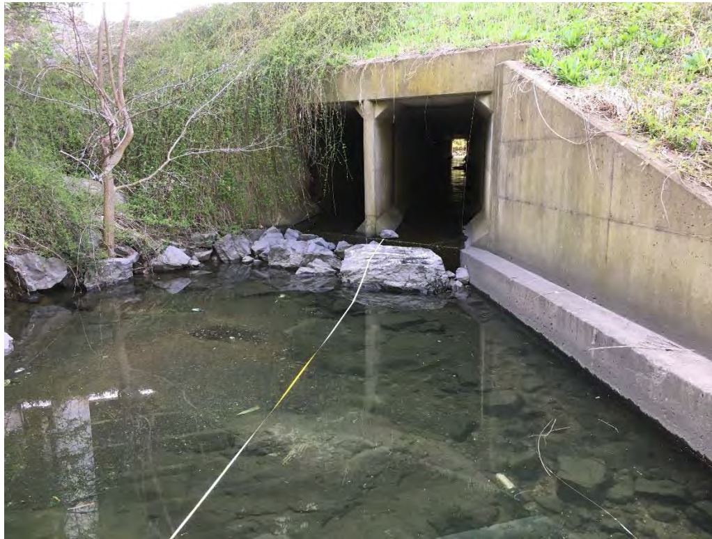
Figure 3-2 Culvert Outfall and plunge pool at the Head of Reach 1
