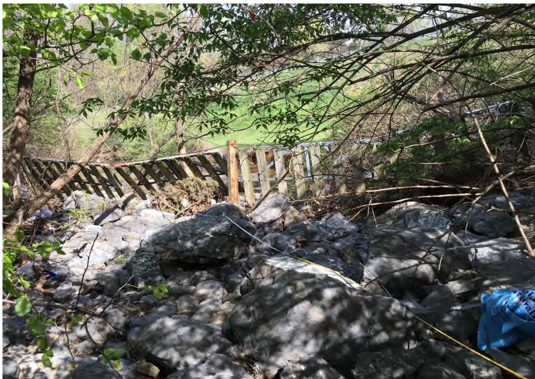
Figure 3-3 Looking Downstream Along Reach 1
