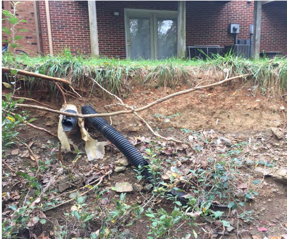
Figure 3-14 Exposed underdrain (9+50)
