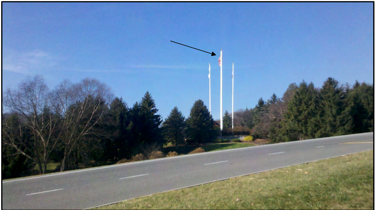
Figure 2: A concealed telecommunications facility as a flagpole at Massanutten Village. 26
