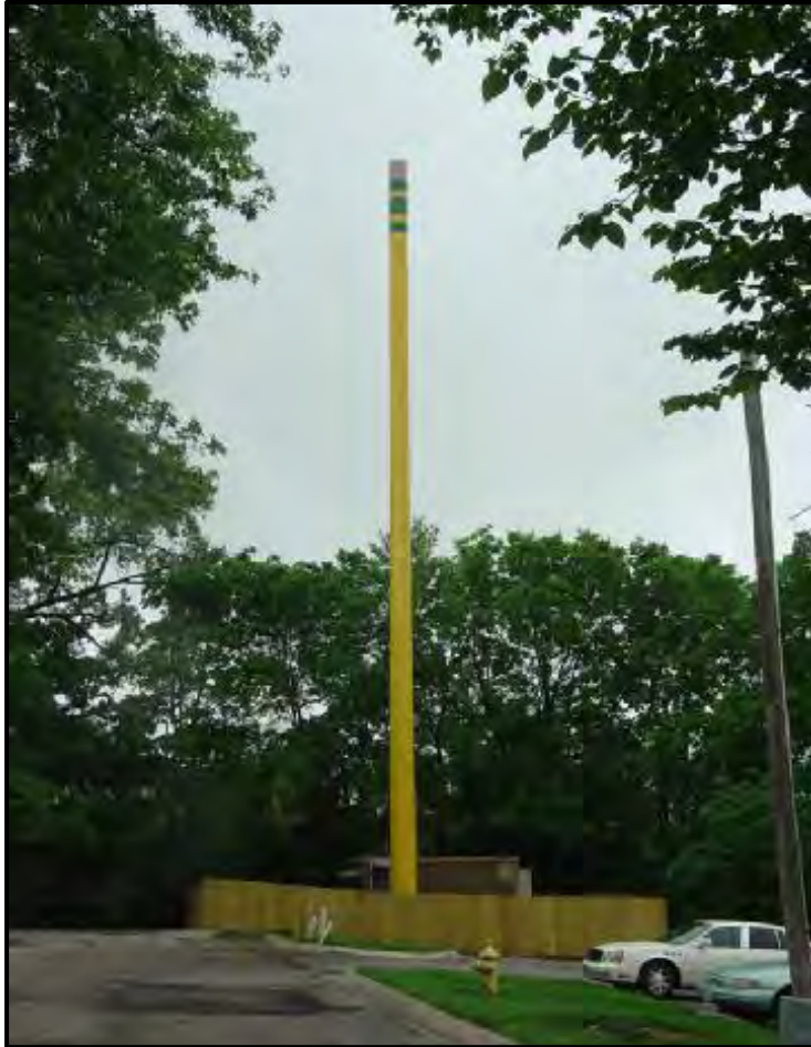
Figure 7: A 100-foot telecommunications tower disguised as a No. 2 pencil located in Liberty, Missouri. 30 City officials hoped the design of the tower would draw attention to the community's commitment to education at institutions such as William Jewel College and the Liberty School District. 31
