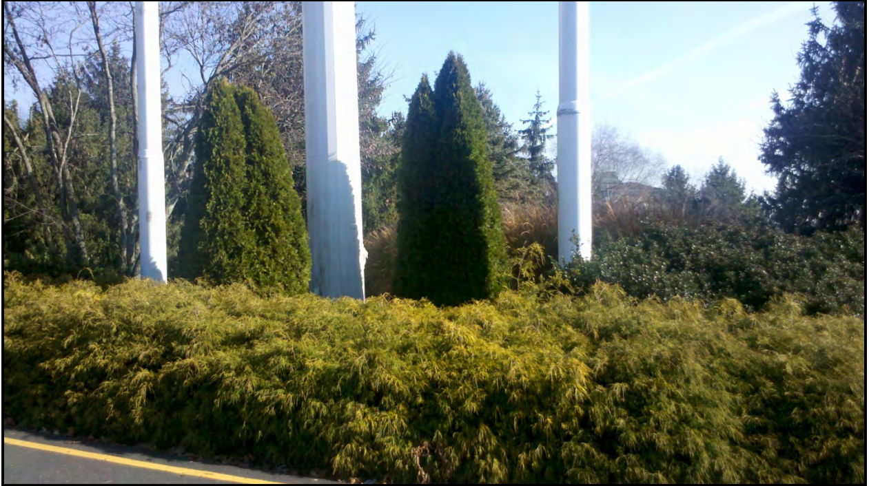
Figure 3: Front view of the base of the concealed telecommunications flagpole. The underground equipment vault is located in the background of the picture, behind the base of the flagpoles. 26
