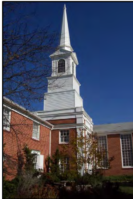
Figure 6: The Unitarian Universalist Church of Roanoke's spire includes telecommunications inside the structure completely concealed from view. 28 The provider, Ntelos, paid to remove the old spire, to install the new spire, and for all of the other necessary equipment. 29
