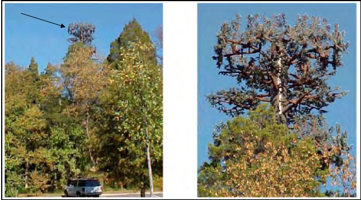
Figure 5: Concealed telecommunications in the form of a tree near Mt. Vernon, VA. 27
